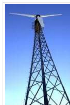
One of two wind turbines built by Anchor Academy students stands tall on the grounds of the old air base north of Havre. The Anchor Academy purchased the land about four years ago.
